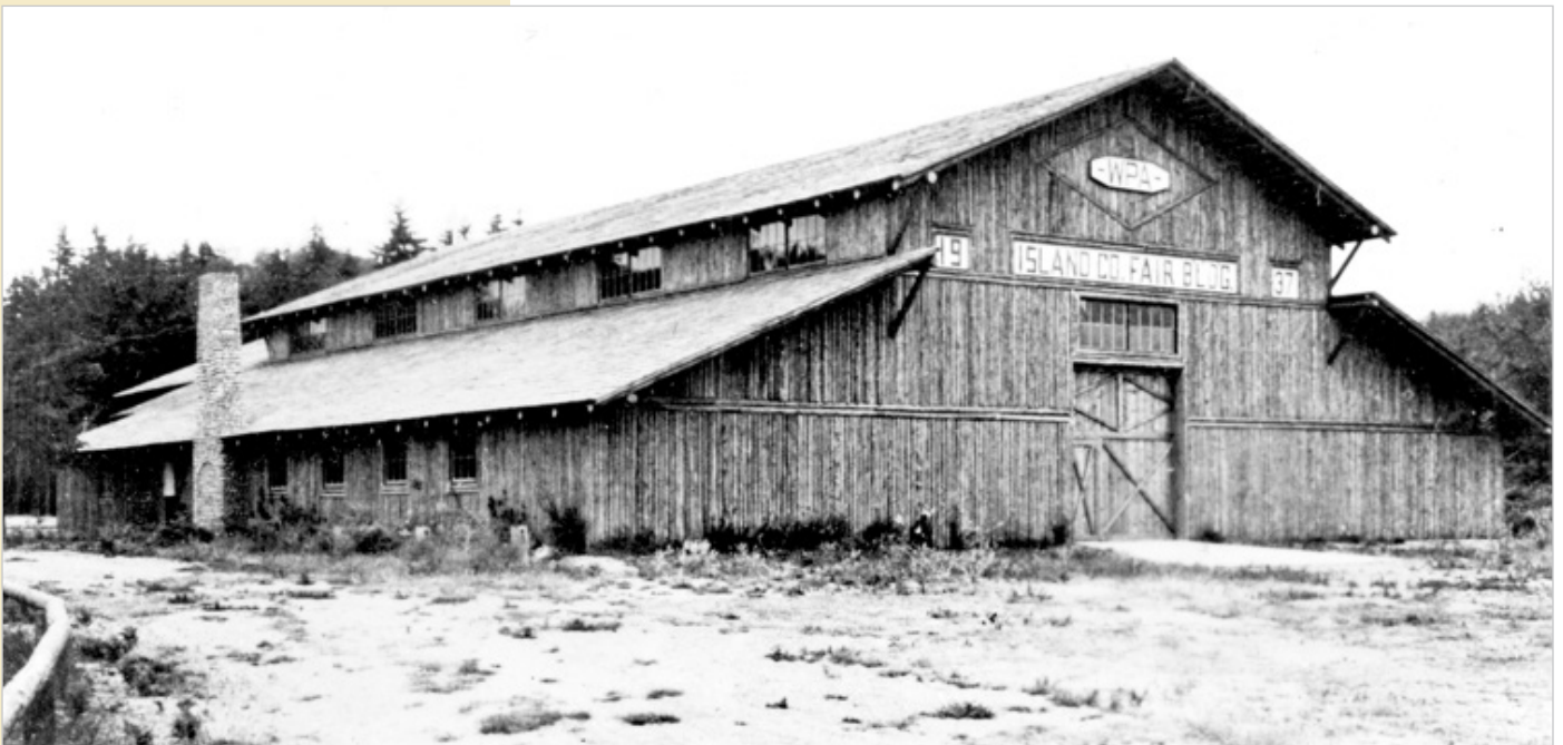
Pole Building circa 1937. Source: courtesy South Whidbey Historical Society
