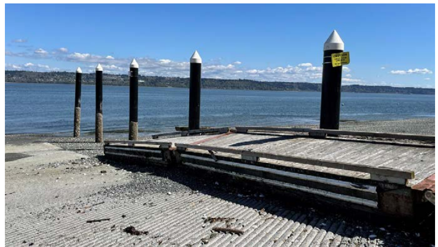
Floating docks along the boat launch are prepared for installation in April after being removed for the winter.
