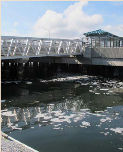
Walkway to Clinton floating pier, prior to removal.
