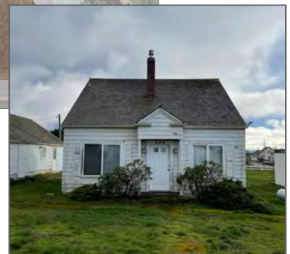
Former on-site manager's house now used for storage.
