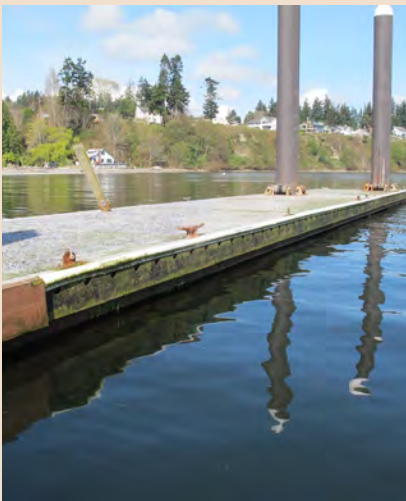
Floating pier at Clinton Dock, prior to removal.
