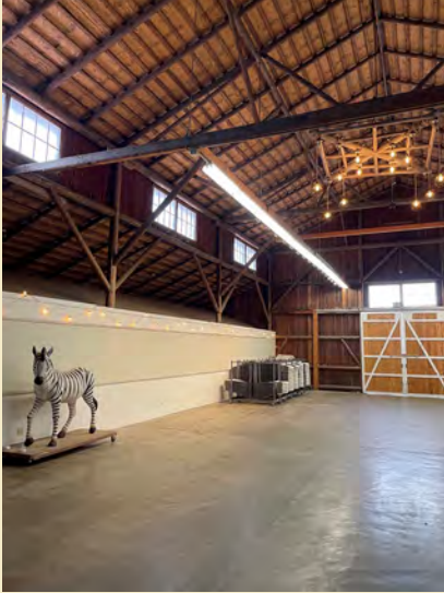
The Pole building is a great event space, but needs additional electrical power and heat.
