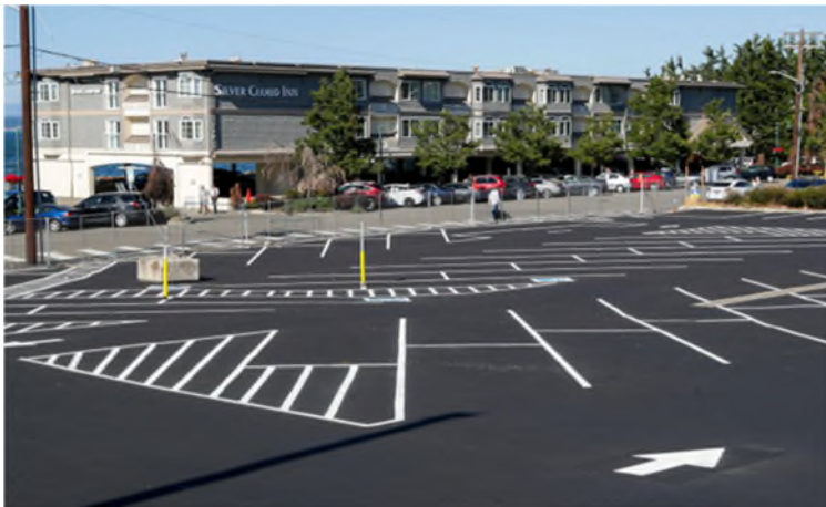
FIGURE 34: MUKILTEO PARKING LOT
