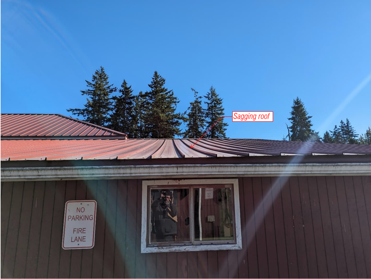
Figure 3 – Sagging Roof
