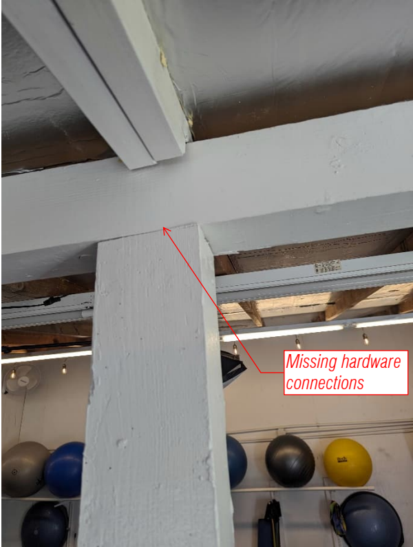
Figure 5 – Lean-to Post and Beam Connection
