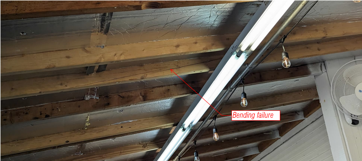
Figure 4 – Failure Rafters
